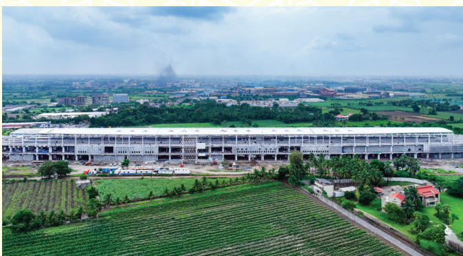
Under Construction Surat Bullet Train Station
