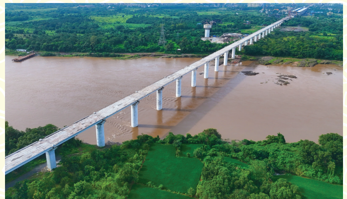
Bridge on Daman Ganga River, Valsad District
