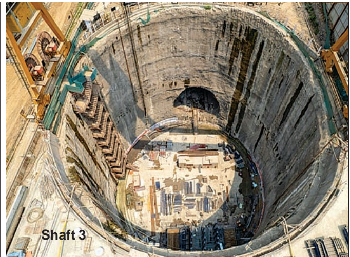
Concrete work for TBM launching in progress, Mumbai, Maharashtra
