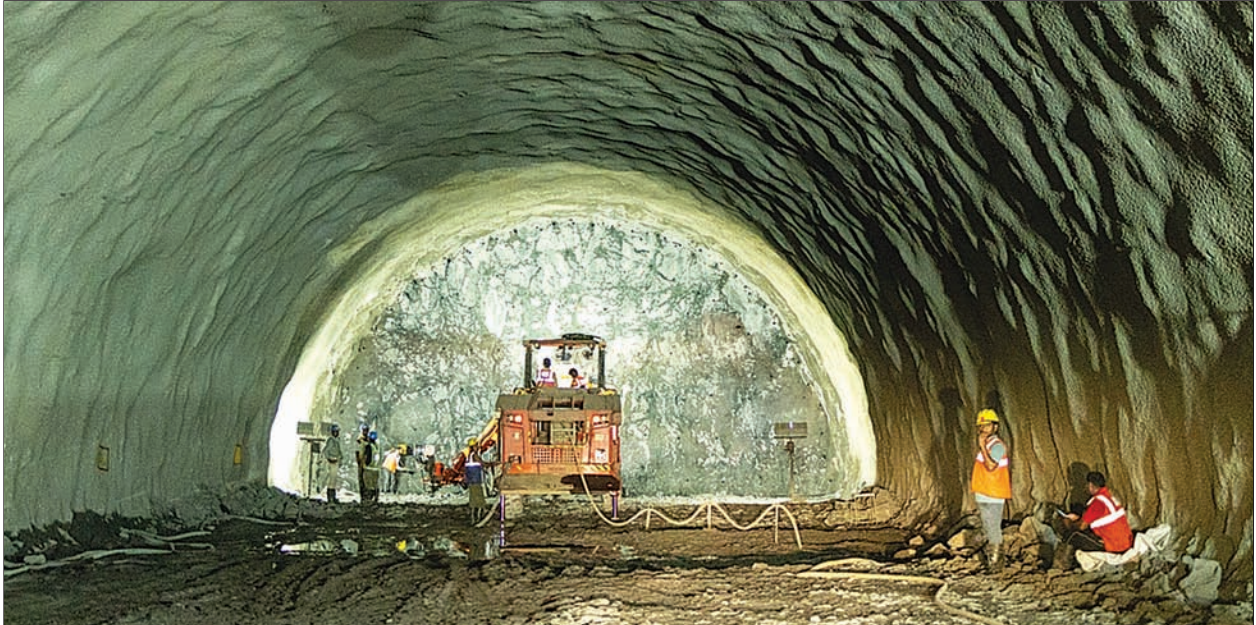
Completion of Main Tunnel excavation (NATM), Thane District, Maharashtra
