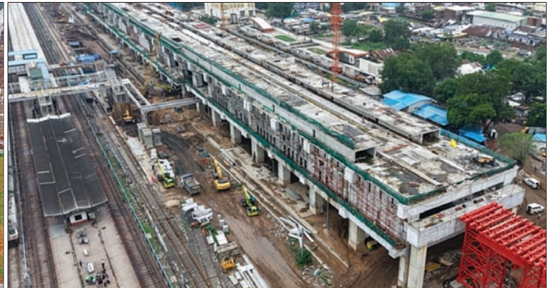
Work in progress at HSR stations, Gujarat
