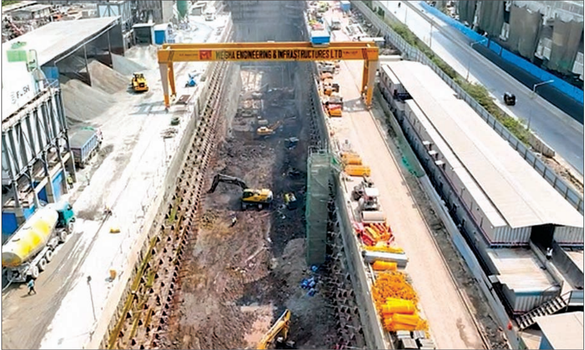
Shaft excavation completed and RCC work in progress, Mumbai, Maharashtra
