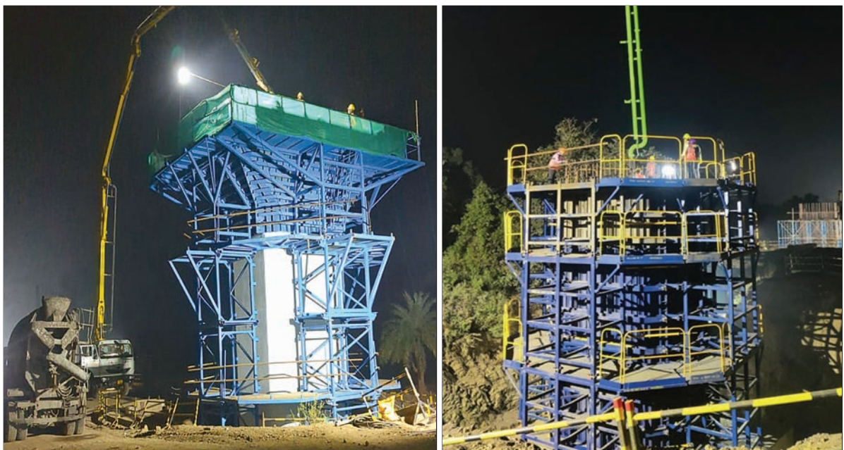
Pier cap and pier casting work in progress, Palghar District, Maharashtra
