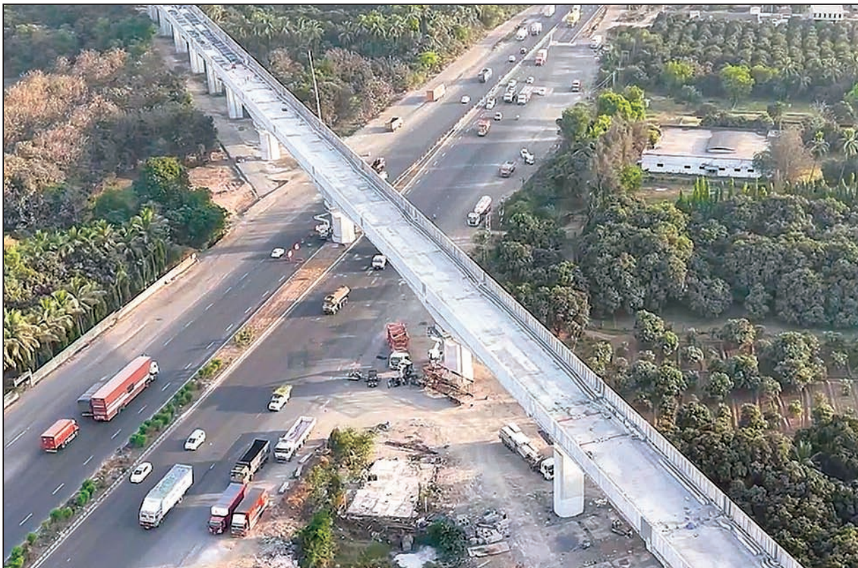
Completion of PSC bridge (GAD – 11), Navsari District, Gujarat
