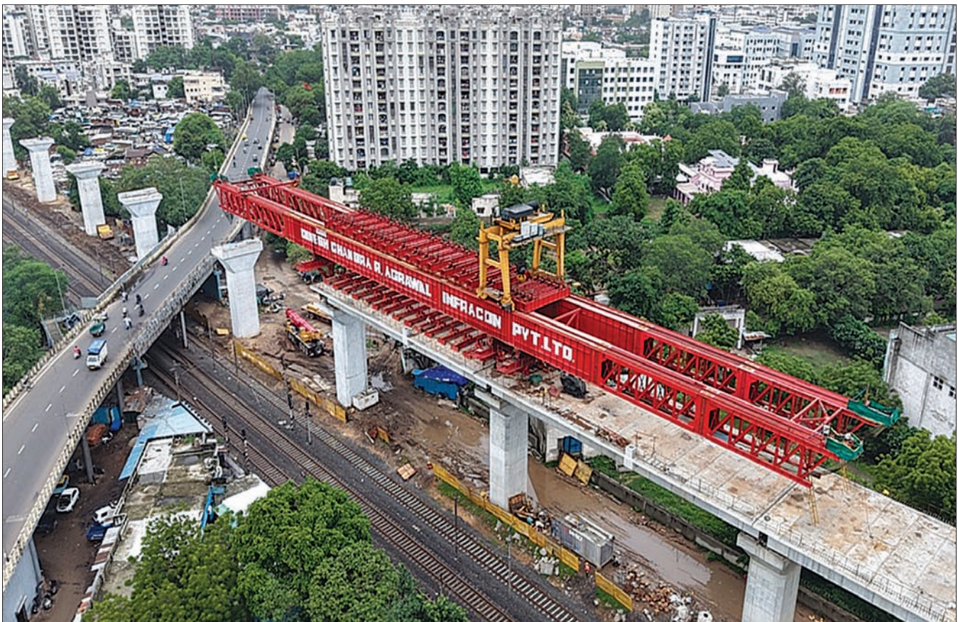
Girder Launching in progress using Segmental Launching Gantry, Ahmedabad District, Gujarat
