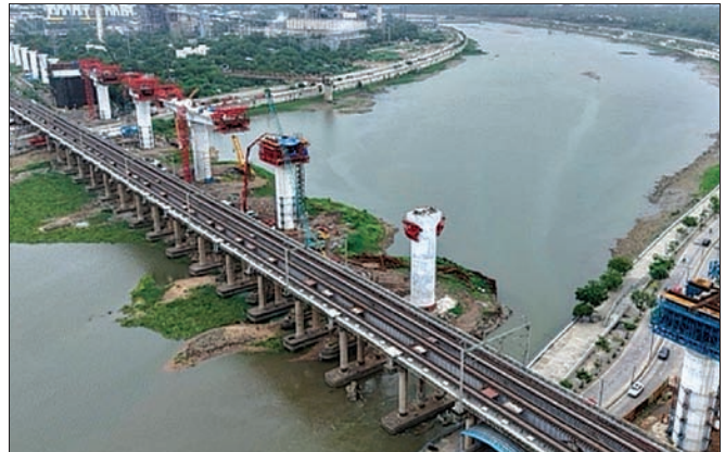
Work in progress at Sabarmati River Bridge, Ahmedabad, Gujarat
