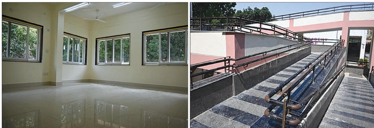
CSR Project – construction of classroom and a ramp, AAD, IIT Roorkee, Uttarakhand
