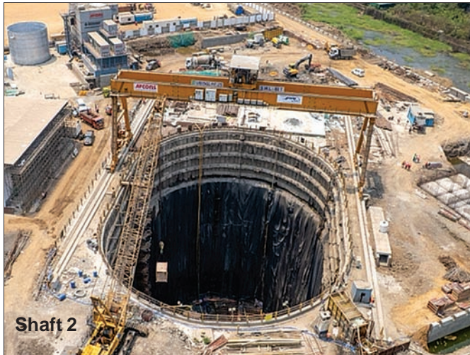
Concrete work for TBM launching in progress, Mumbai, Maharashtra
