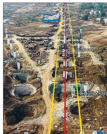
Construction of viaduct in progress, Thane District, Maharashtra
