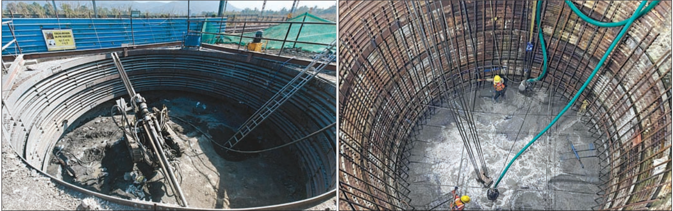
Shinsho Pile work in progress, Palghar, Maharashtra
