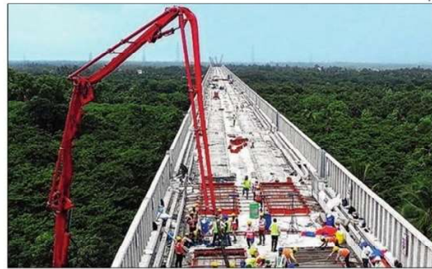
It is for the first time that the J-slab ballastless track system, a feature of Japan's high-speed rail system Shinkansen, is being used in India
