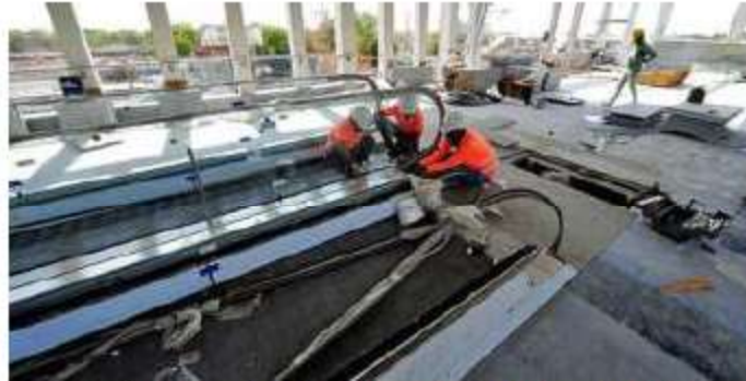
Contracts for the track works in the entire Gujarat section of the project have been awarded. FILE PHOTO
