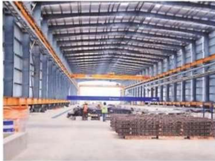
The Track Slab Manufacturing Facility is fully automated.
