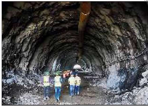
The 350-metre long tunnel has a diameter of 12.6 metres
