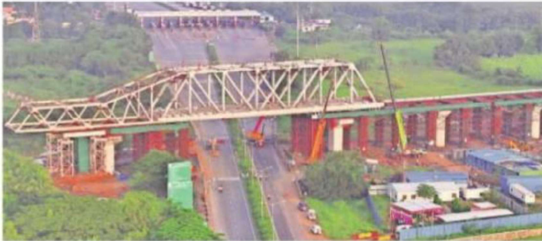
The steel bridge is located near Kamrej Toll Plaza Express
